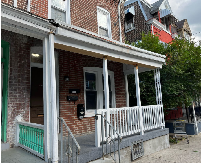
Porch following replacement of the posts and railings, 2023. (Applicant)
