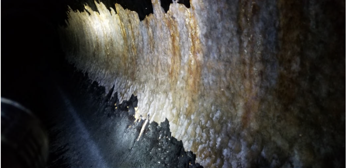
Figure 18- ARV 5 toward 6 - Coating disbondment and ½" mortar loss along springline, rust pattern from steel shell beginning to seep through mortar following wire pattern
