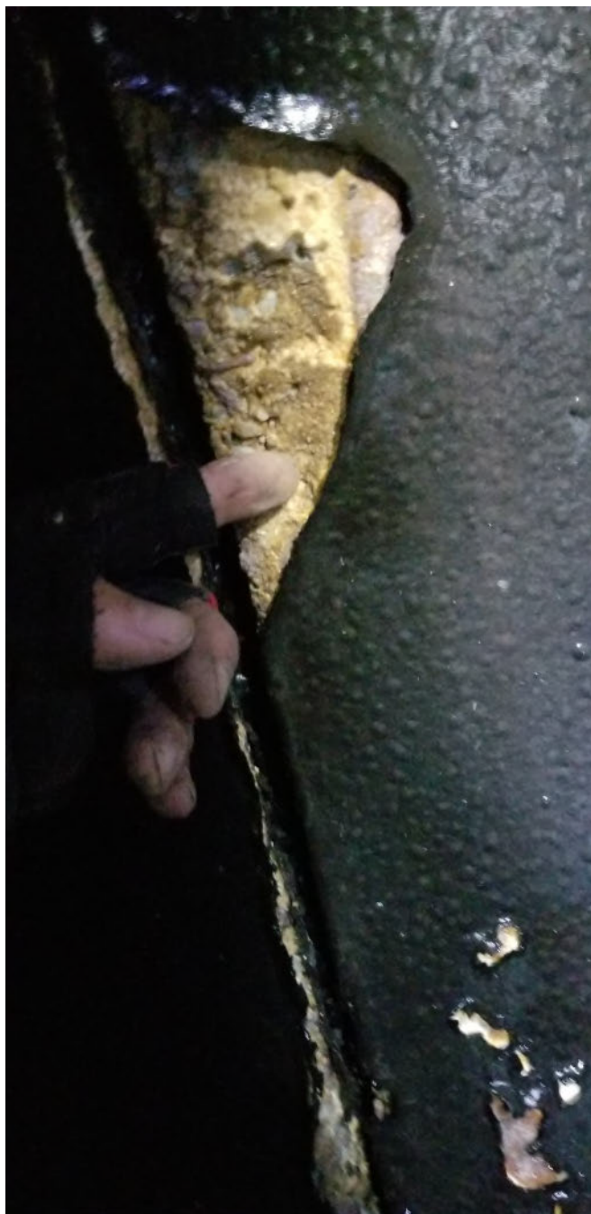
Figure 15 - ARV 5 toward ARV 6 - Coating disbondment at joint
