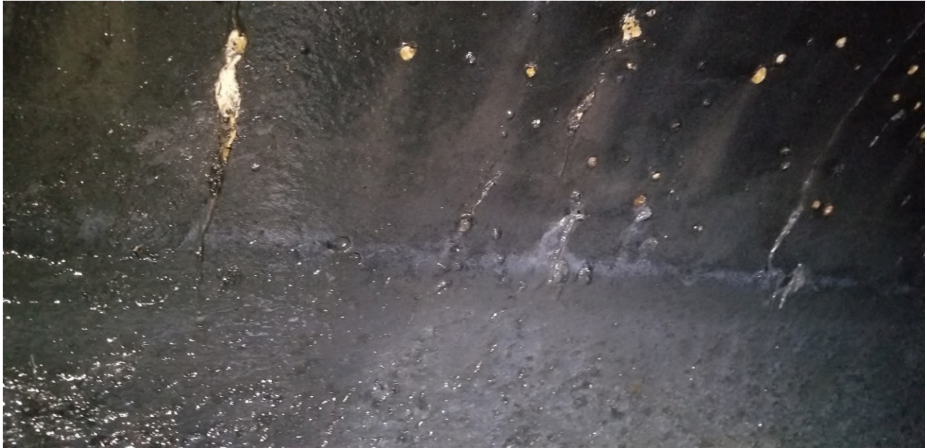
Figure 11 - ARV 5 toward ARV 4 - 20' Upstream - Cracking of coating and exposure of underlying mortar
