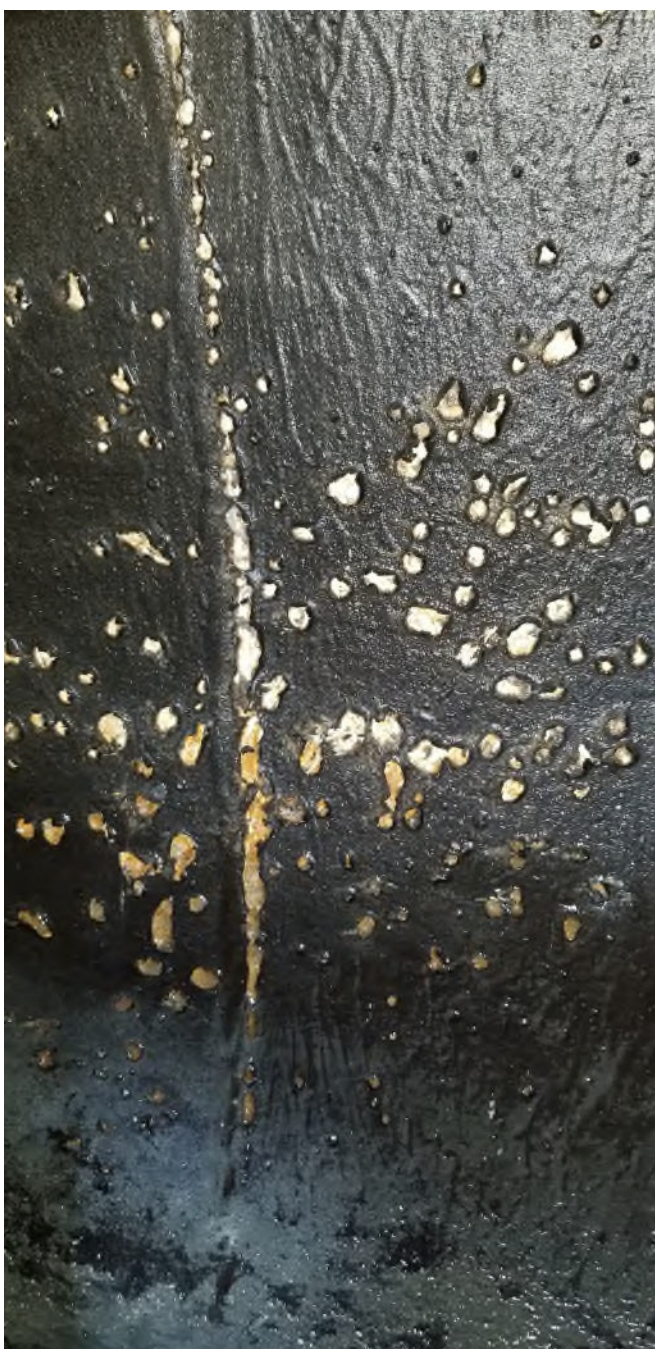
Figure 22 - ARV 6 toward ARV 5 - Coating Blisters and Disbondment
