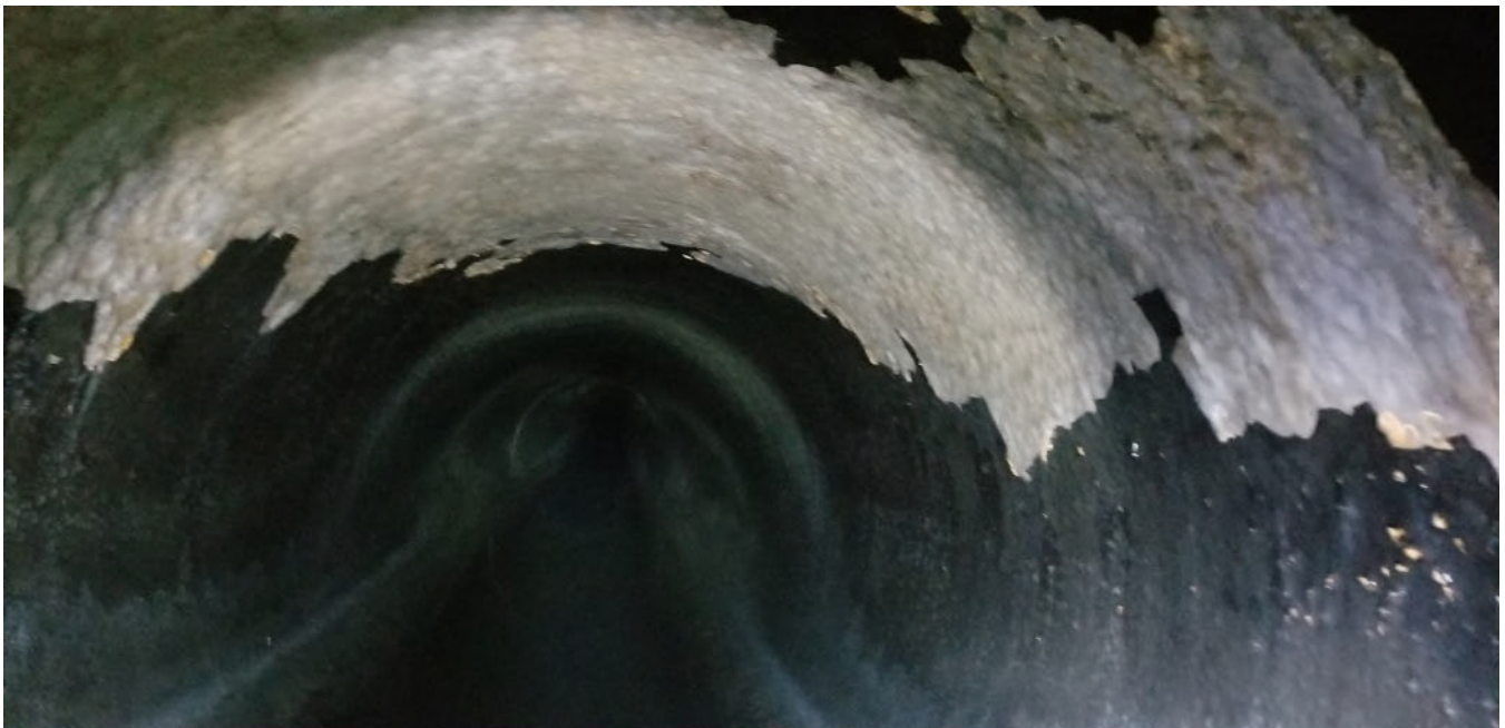
Figure 19- ARV 5 toward 6 - Coating disbondment and 3/8" mortar loss springline to springline
