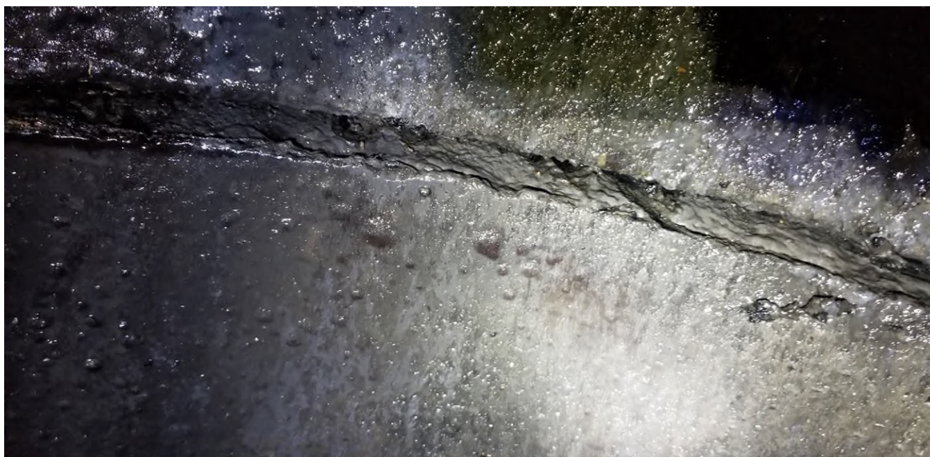
Figure 7 - ARV 5 toward ARV 4 - Unmudded joint
