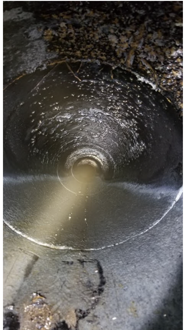
Figure 28 - ARV 8 toward ARV 9 - Blisters in Coating
