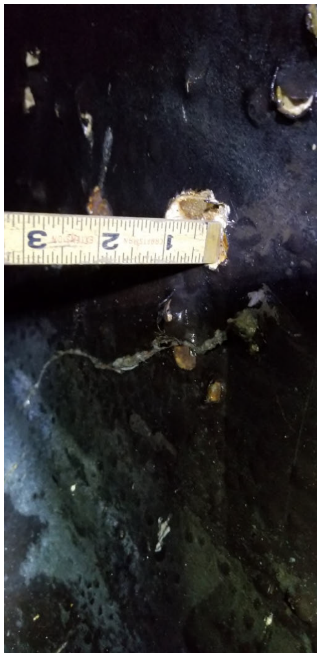
Figure 14 - ARV 5 toward ARV 6 - H 2 S attack at coating blister
