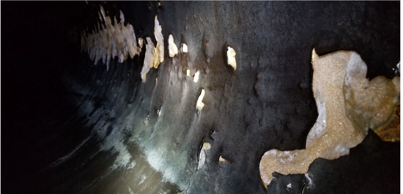
Figure 17 - ARV 5 toward 6 - Coating disbondment along springline with 1/2" mortar loss under blisters
