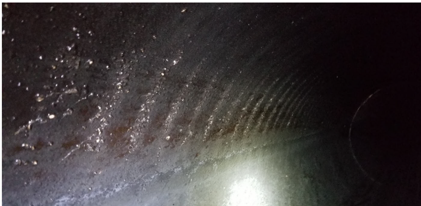
Figure 8 - ARV 5 toward ARV 4 - 8' Upstream - Disbonding of coating along spray pattern
