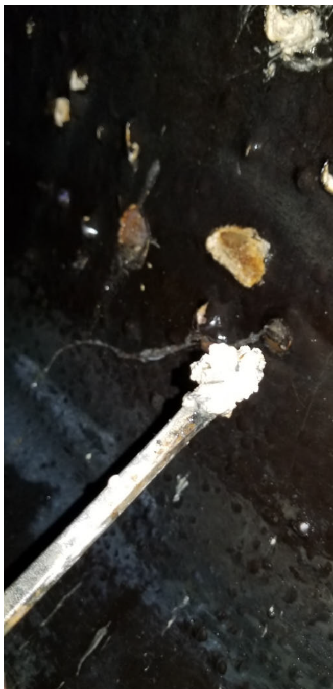
Figure 12 - ARV 5 toward ARV 6 - Gypsum from H 2 S attacked mortar
