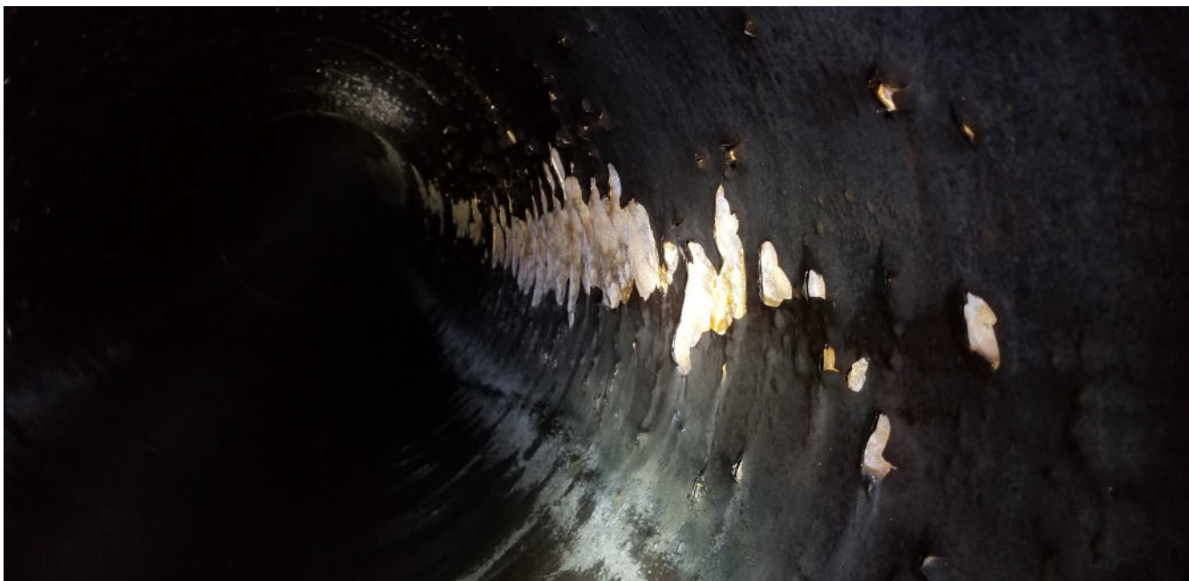
Figure 16- ARV 5 toward 6 - Coating disbondment along springline following wire pattern
