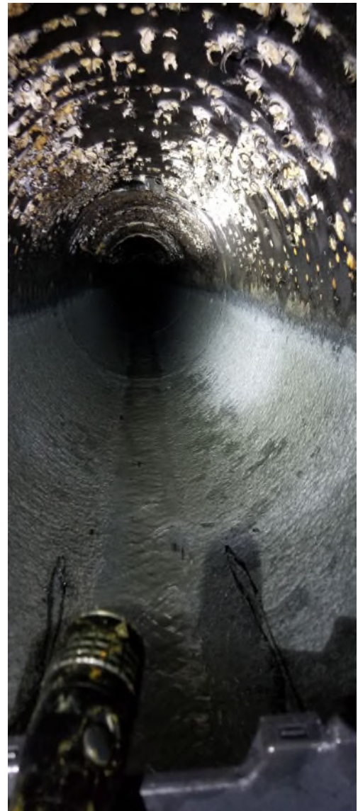
Figure 25 - ARV 8 toward ARV 7 - Blisters in Coating
