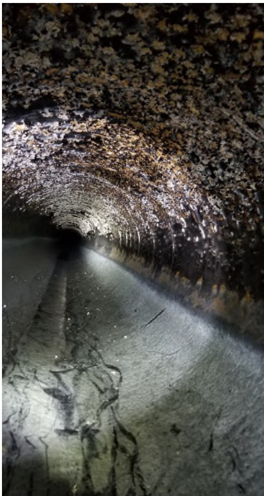
Figure 26 - ARV 8 toward ARV 7 - Blisters in Coating
