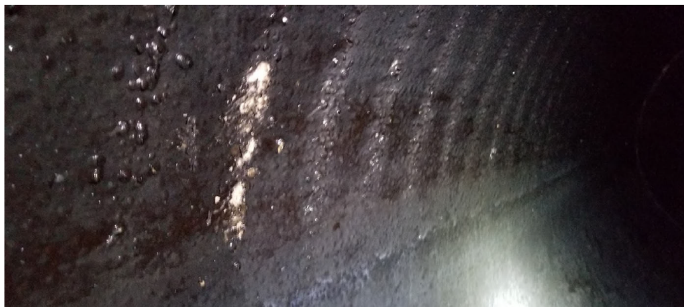
Figure 10 - ARV 5 toward ARV 4 - 8' Upstream - Soft mortar revealed under the disbonded coating (typ)
