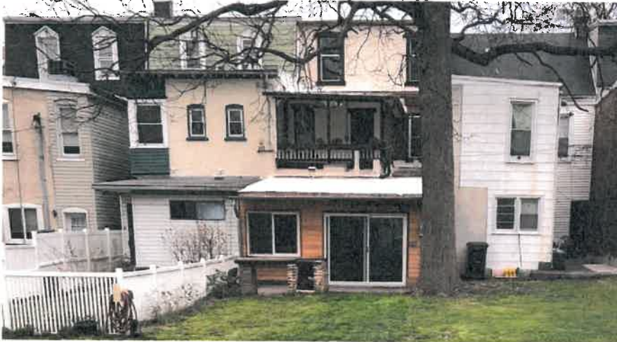
Rear Facade and Adjacent Properties (Applicant)
