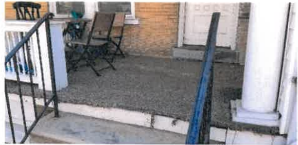
Porch Floor Decking (Applicant)
