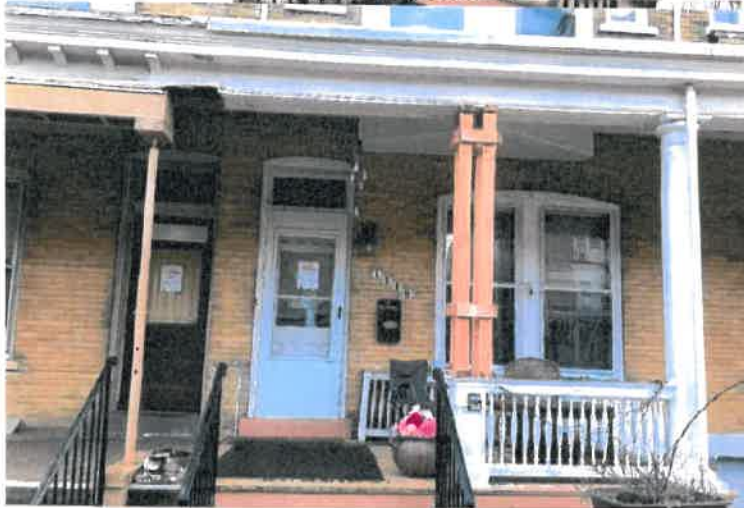
Primary Façade (Applicant)
