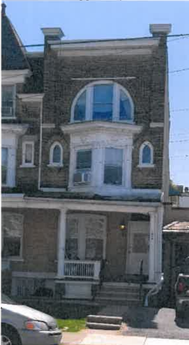
Primary Façade, view looking south (Applicant)
