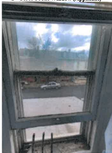
2 nd Floor Front Window (Applicant)
