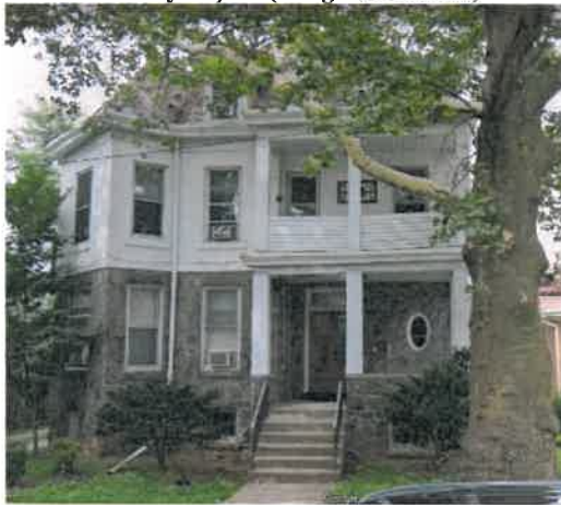
Primary Façade (Google Streetview)
