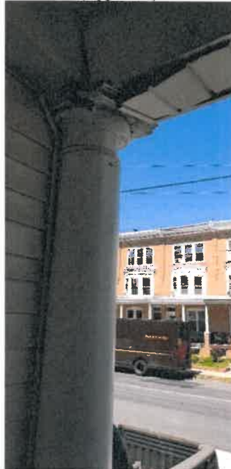
Porch Column and Header (Applicant)
