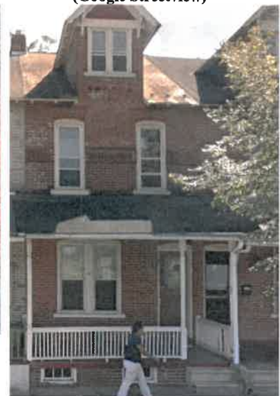
Primary Facade, 2019 (Google Streetview)
