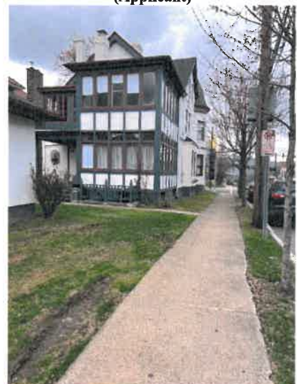
Rear facade, view from Linden St. (Applicant)
