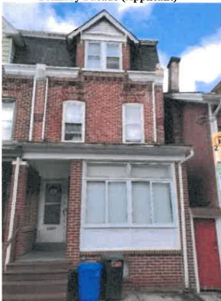
Primary Facade (Applicant)
