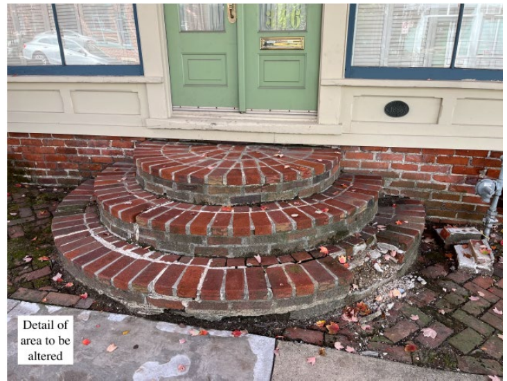
Existing steps at 346 N. 8th Street. (Applicant)
