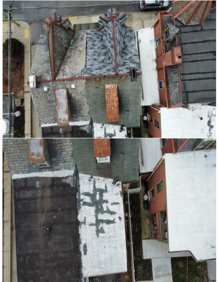
Current roof condition (applicant)
