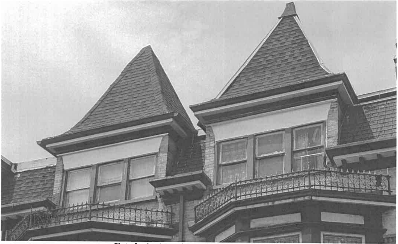
Photo showing the capping installed over the lintels, 2023. (HARB files)
