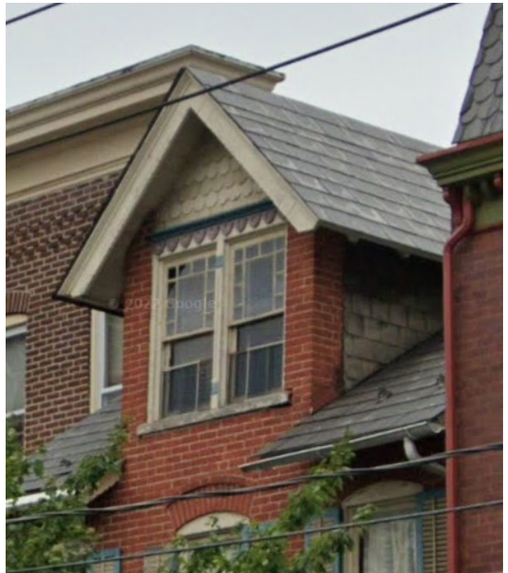
Detail of roof, 2019. (Google StreetView)
