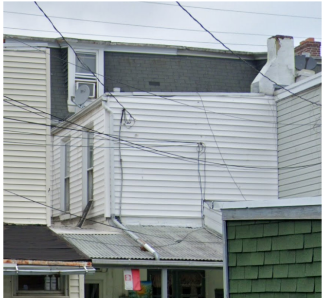
Rear of Property, 2019 (Applicant)
