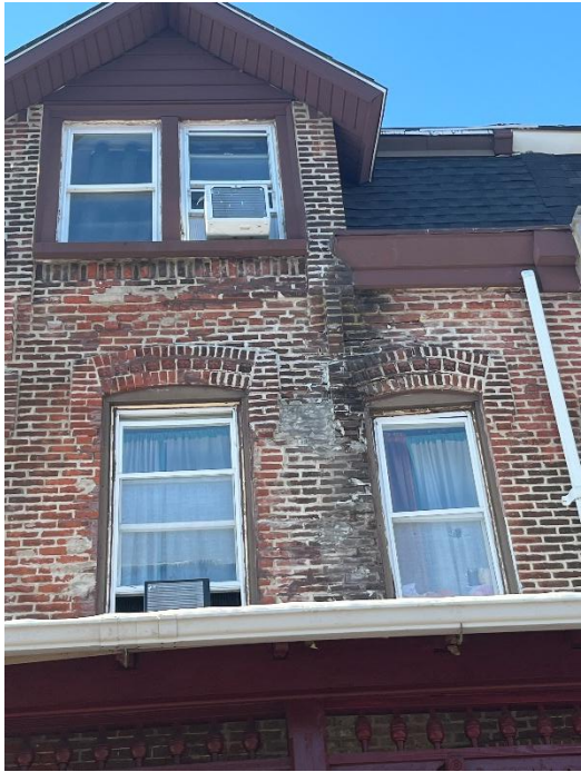
Existing Upper Floor Condition (Applicant)
