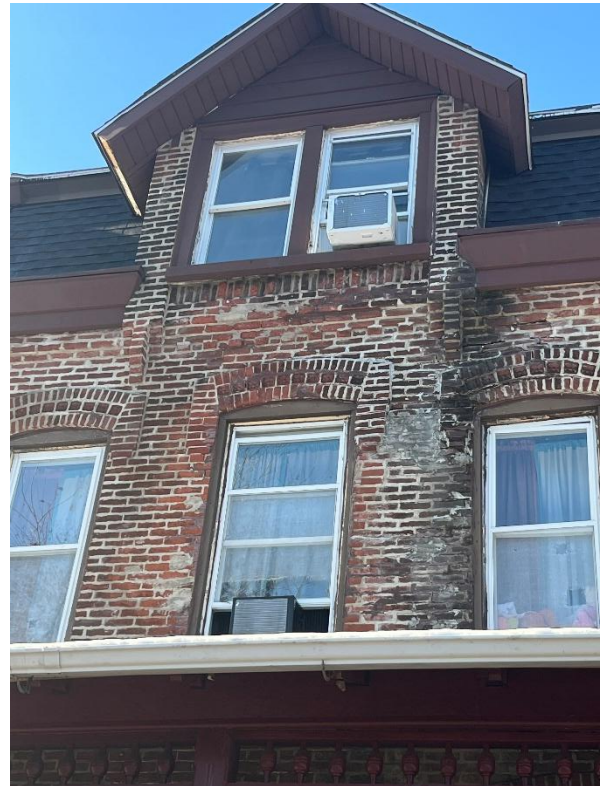
Existing Upper Floor Condition (Applicant)
