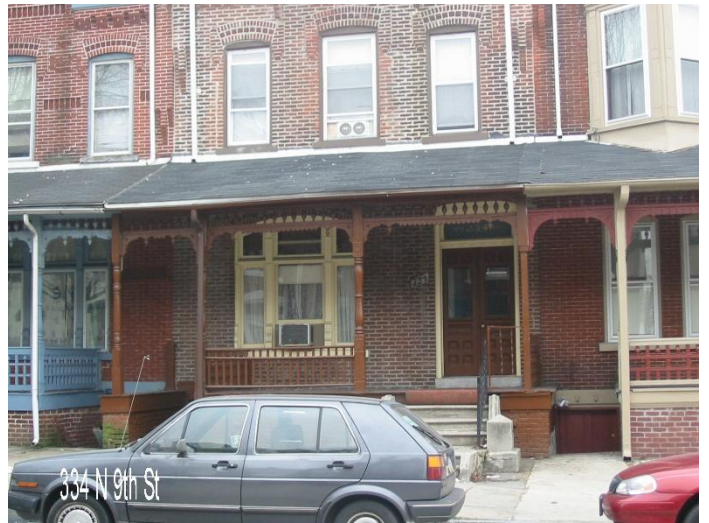
Existing Condition (Applicant)
