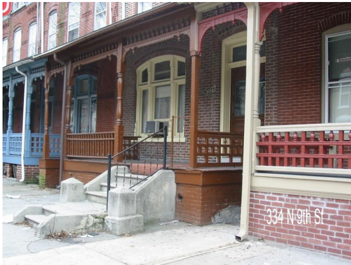
Existing First Floor Condition (Applicant)
