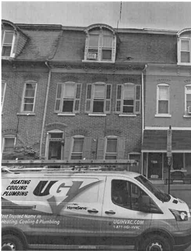
Front Elevation (Google Street View)
