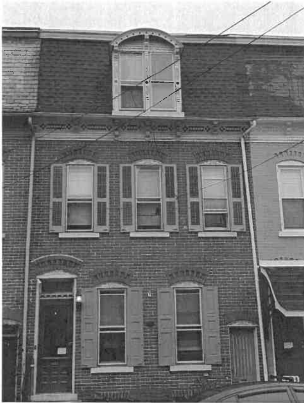
Repaired Roof Close-Up (Applicant)
