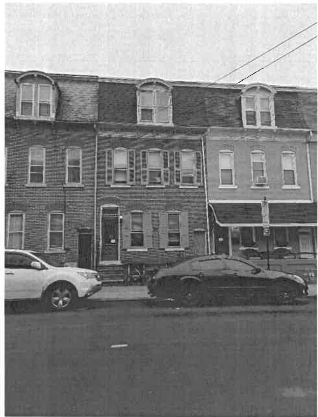
Repaired Roof (Applicant)
