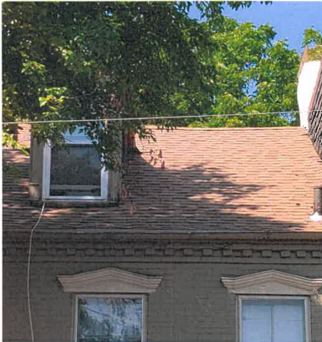
Front Roof Aerial of 213 N. 11th Street, 2023. (HARB files)
