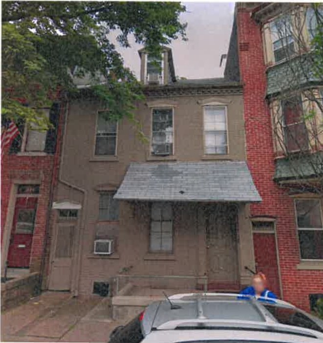
Front façade of 316 N. 8th Street before reroofing, 2019. (Google StreetView)
