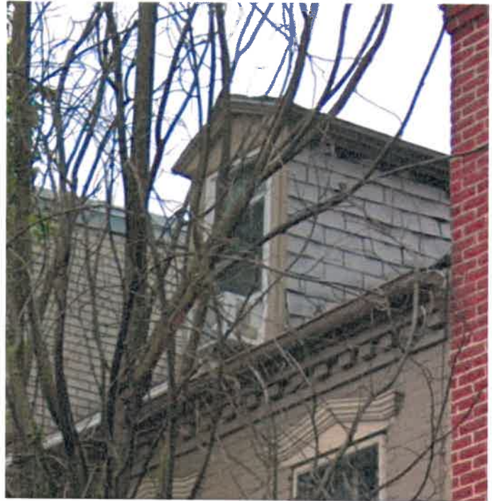
Dormer of 316 N. 8th Street before refoofing, 2019. (Google StreetView)
