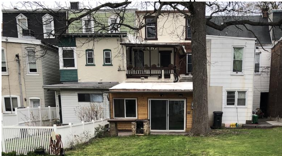
Rear Facade and Adjacent Properties (Applicant)
