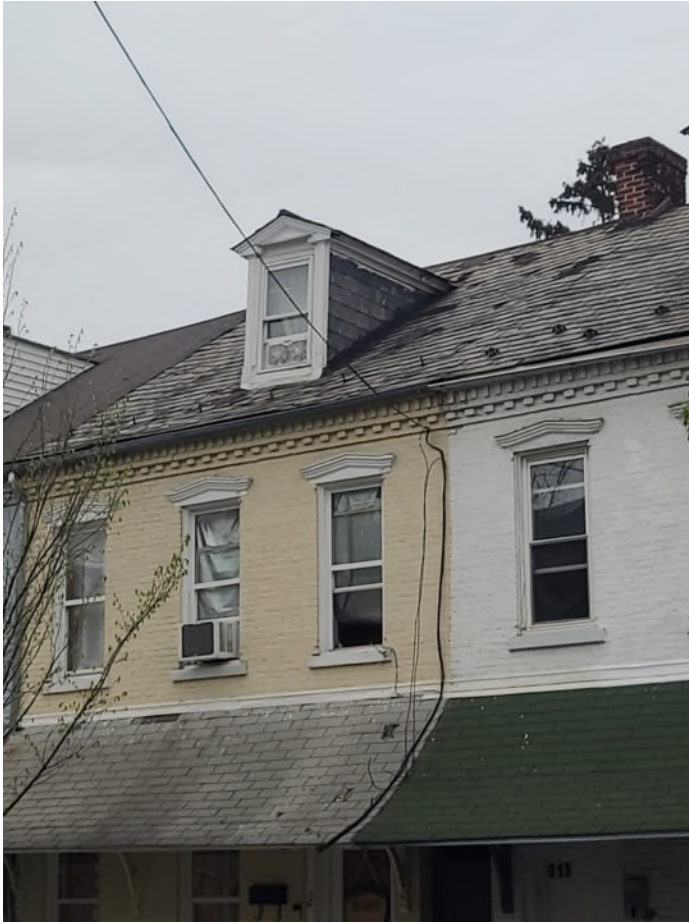
Current Roof (Applicant)
