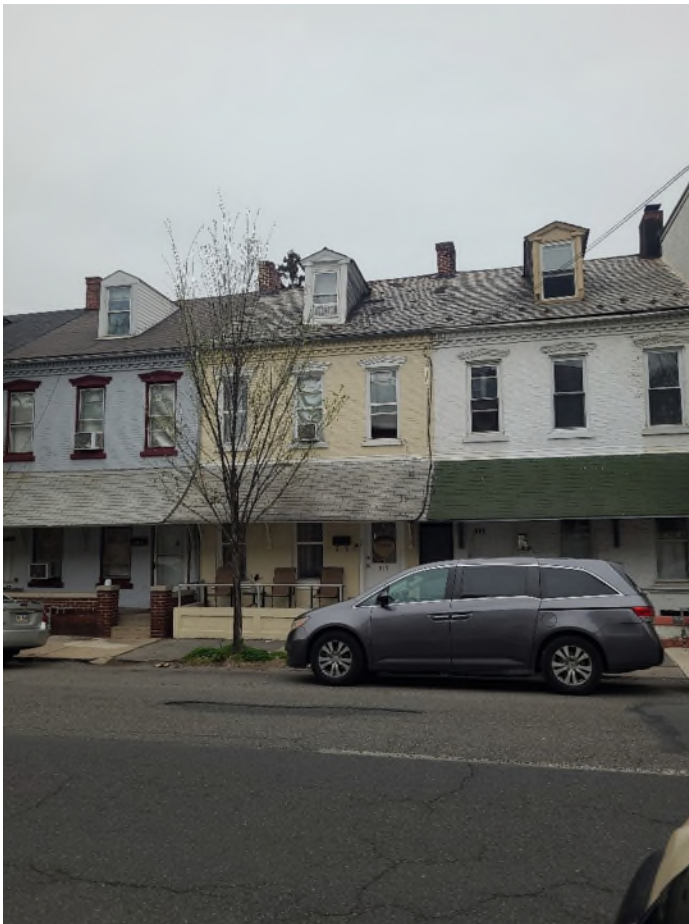
Current Roof (Applicant)
