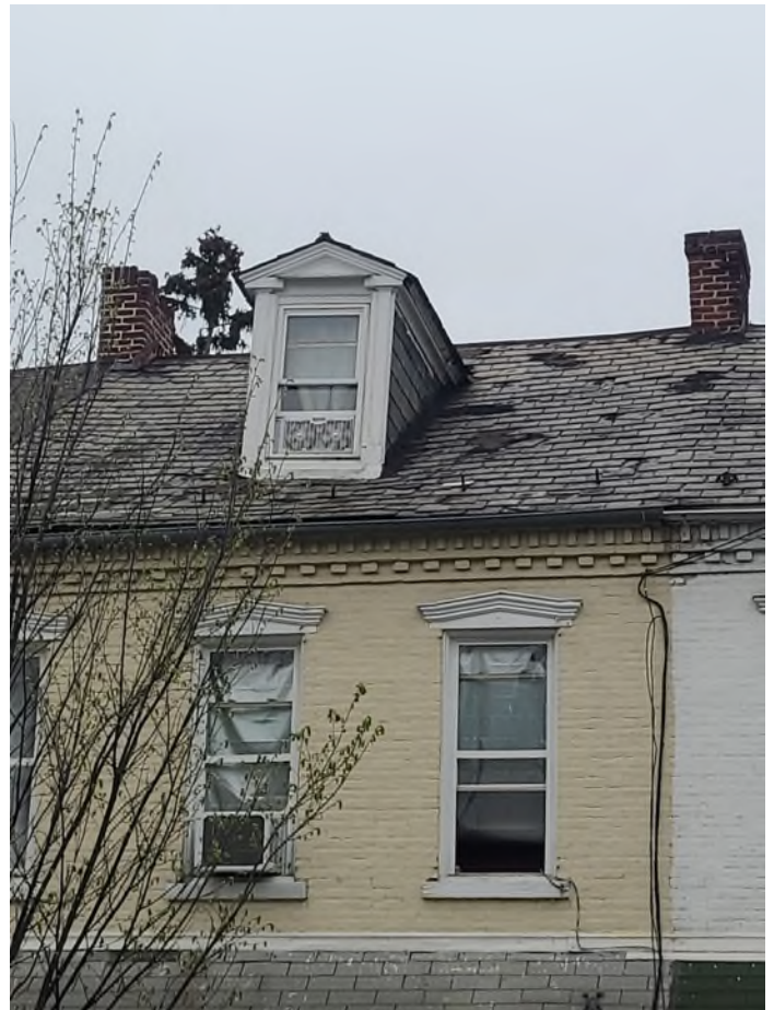
Current Roof (Applicant)
