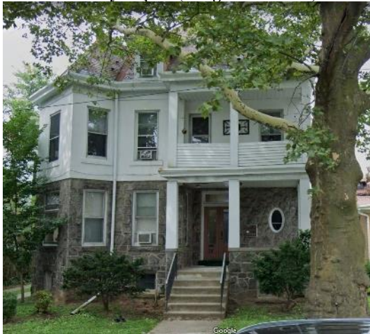
Primary Façade (Google Streetview)
