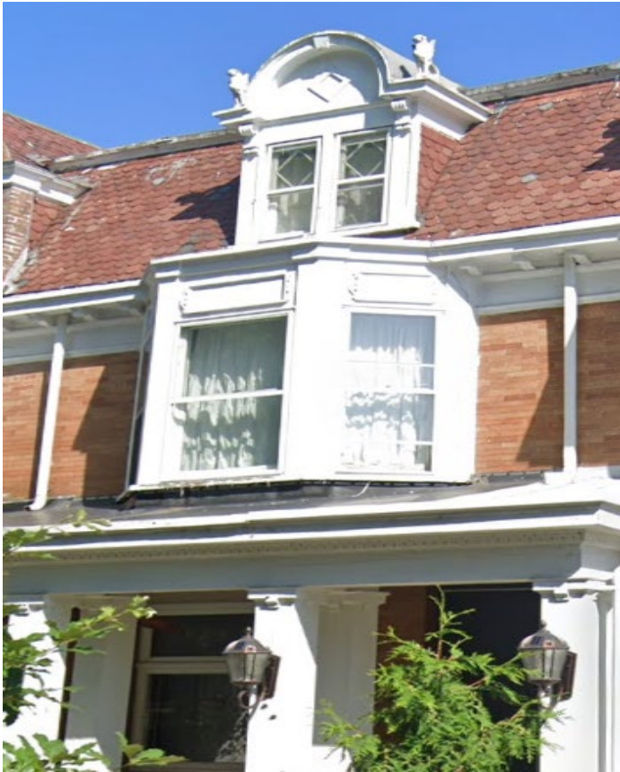
Front façade of 1529 W. Street, 2023. (Google Street View)
