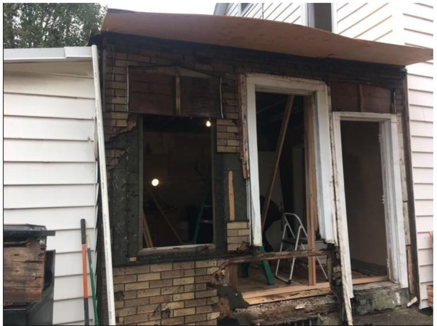
Photo of the rear ell following the removal of the siding. (HARB files)
