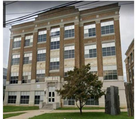
with flat-head bolts which are visible on the exterior surface. The metal panels and cast-iron pieces have all deteriorated, are loose, falling and past their useful life. The proposed work includes removal of the deteriorated applied cast iron trim and install new fypon panels fabricated to matching existing details.
