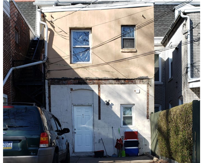
Rear of 141 N. 10 th Street following removal of the porch roof, 2023. (HARB files)
