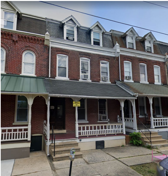
Front façade of 141 N. 10 th Street, 2023. (Google StreetView)
