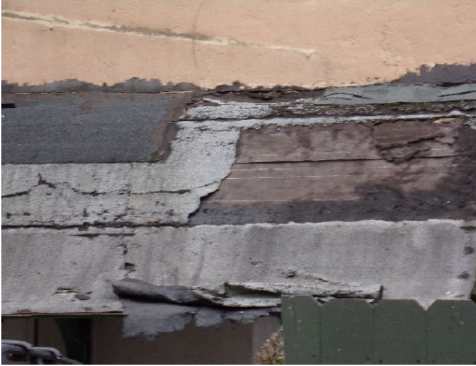
Detail of porch roof prior to removal. (Applicant)
