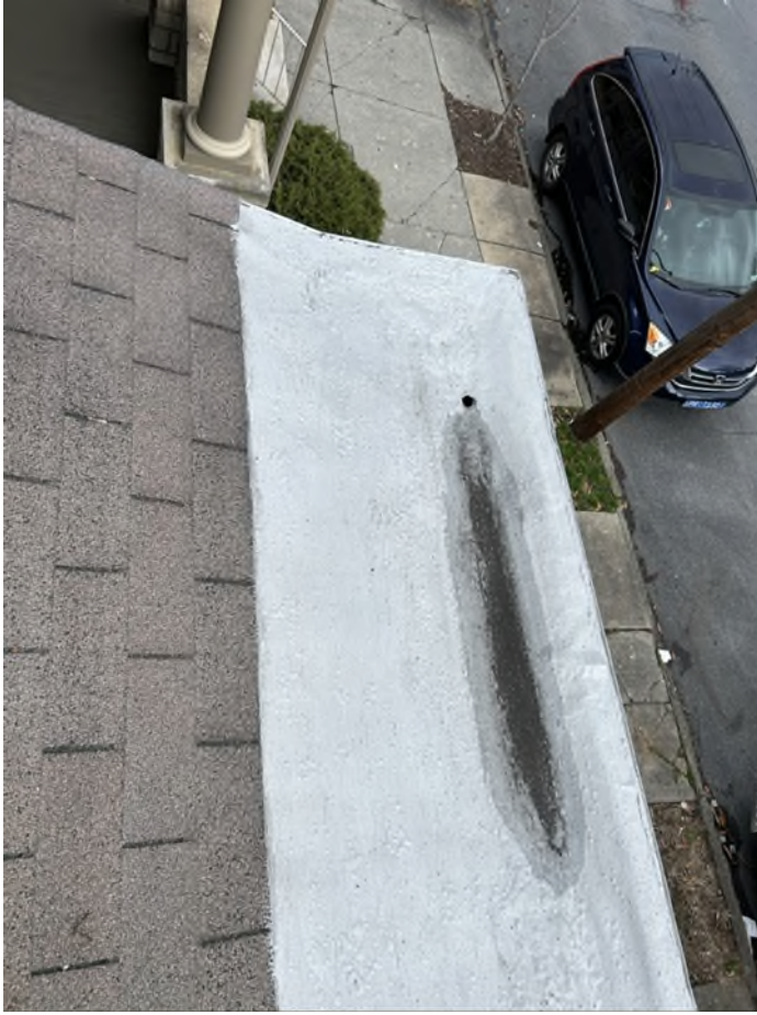
Current Porch Roof (Applicant)
