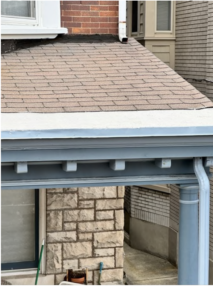
Current Porch Roof (Applicant)
