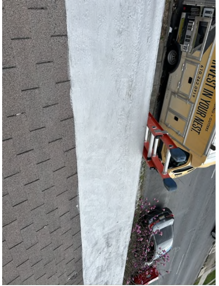
Current Porch Roof (Applicant)
