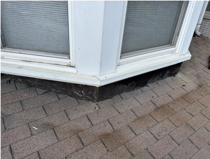
Roofing at Bottom of Bay Window (Applicant)
