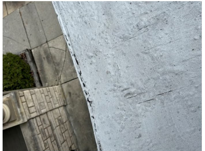
Current Porch Roof (Applicant)
