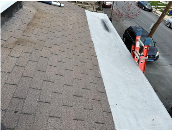
Current Porch Roof (Applicant)
