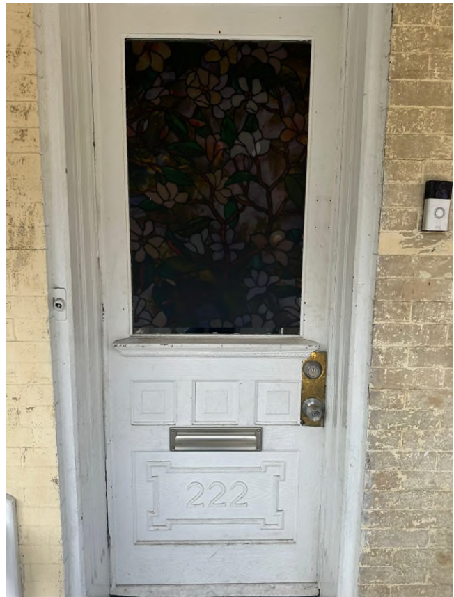
Existing Door (Applicant)
