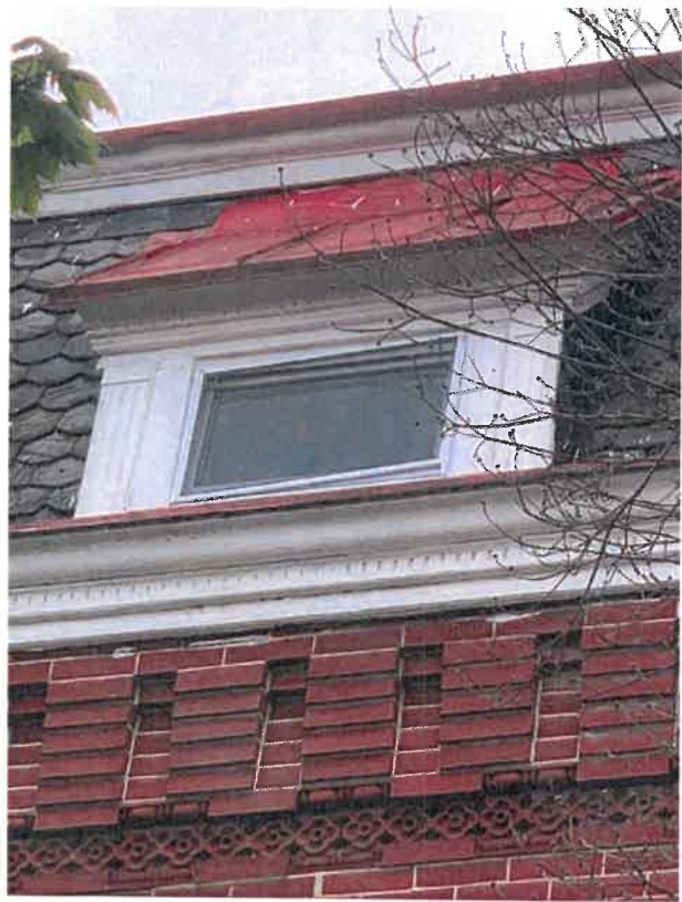
Installed Third Floor Window (Applicant)
