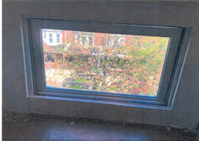
Installed Third Floor Window (Applicant)
