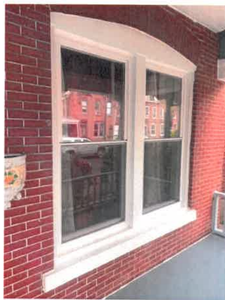
Installed First Floor Windows (Applicant)
