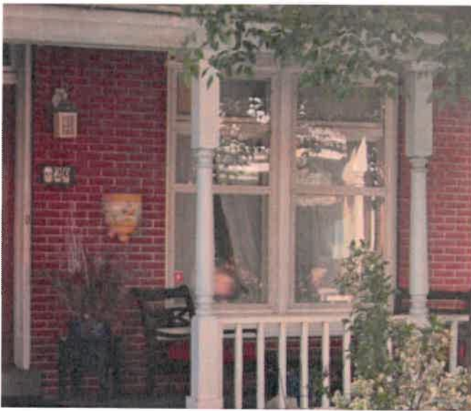
Previous First Floor Windows, c.2019 (Google)
