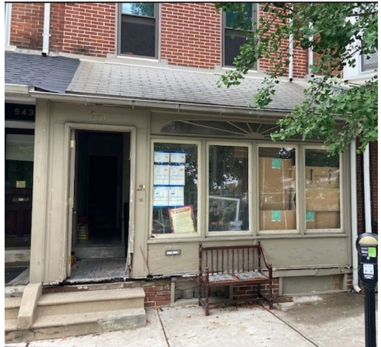
The enclosed porch at 941 W. Turner Street. (Applicant)
