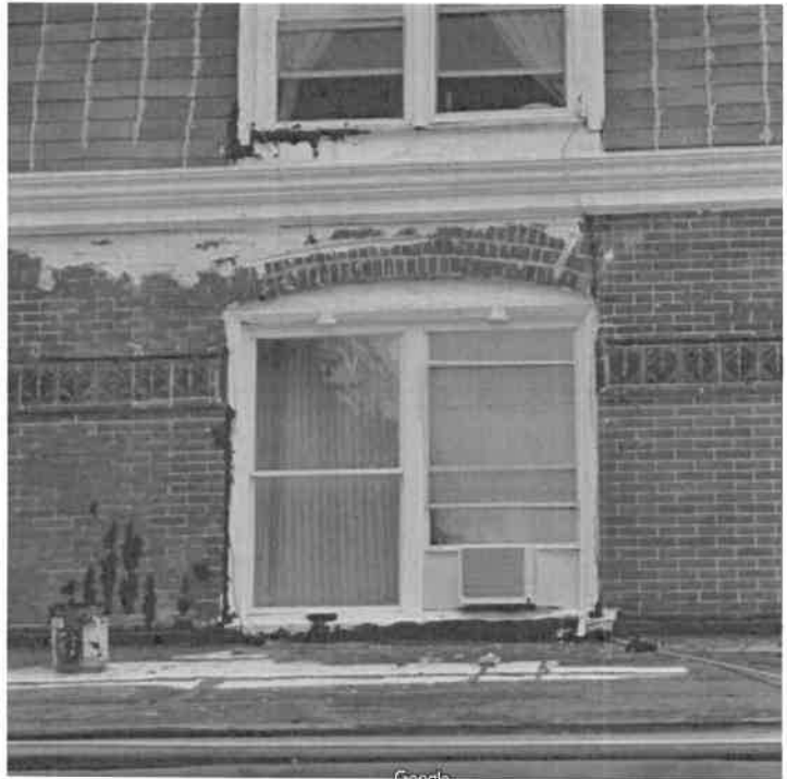
Photo showing the windows and framing to be replaced. (Google StreetView)
