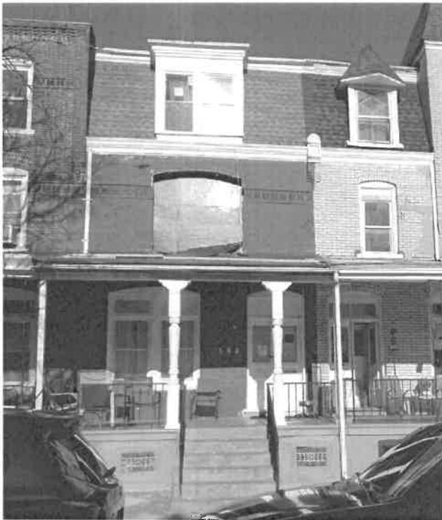
Front façade with windows removed and boarded, 2023. (Applicant)
