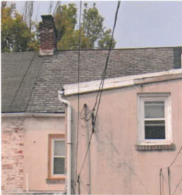
Rear view of 515 N. Park Street, 2023. (Google StreetView)
