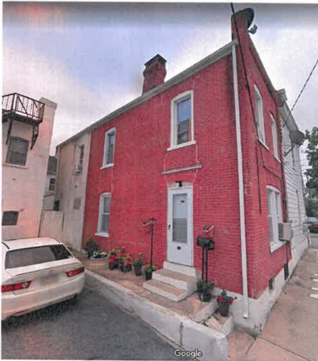
Front and side façades of 327 N. Nagle Street, 2019. (Google StreetView)
