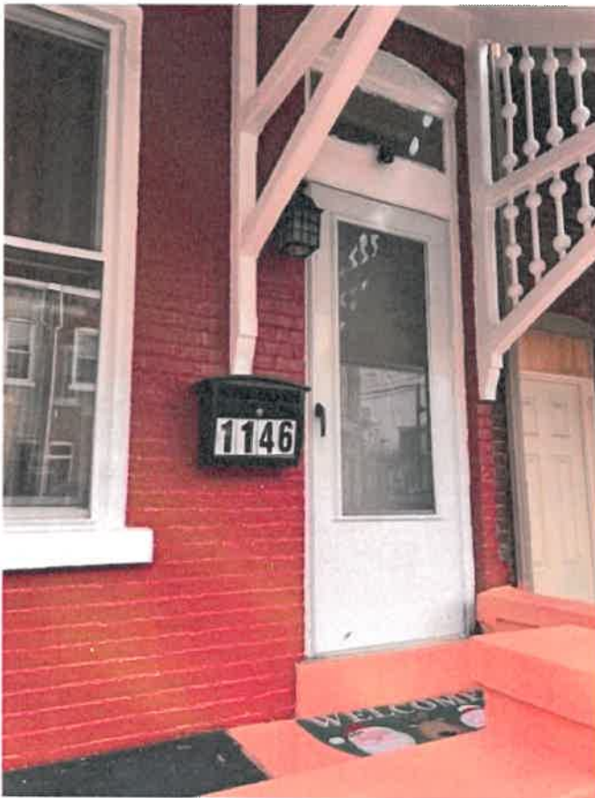
1146 W. Turner Street, 2023. (Applicant Image-Storm Door)
