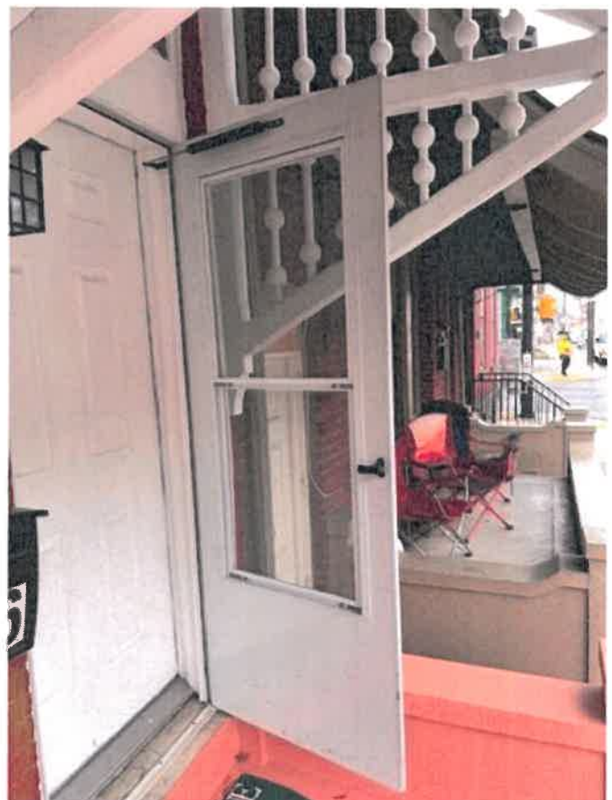
1146 W. Turner Street 2023. (Applicant Image-Front Entry Door)
