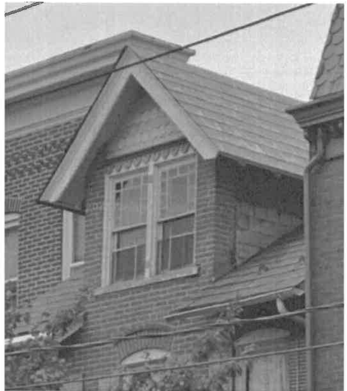
Detail of roof, 2019. (Google StreetView)
