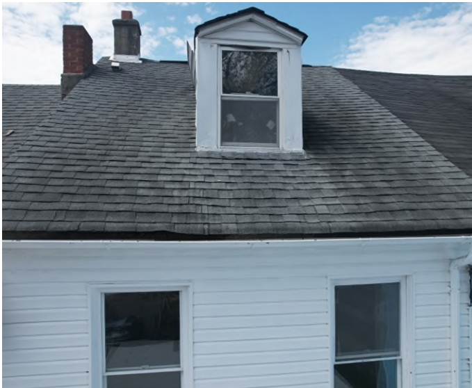
Current Roof (Applicant)
