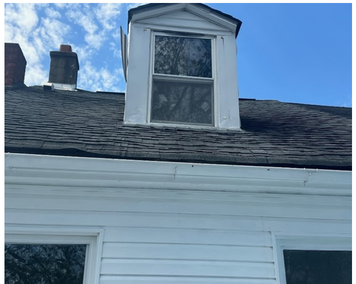
Current Roof (Applicant)
