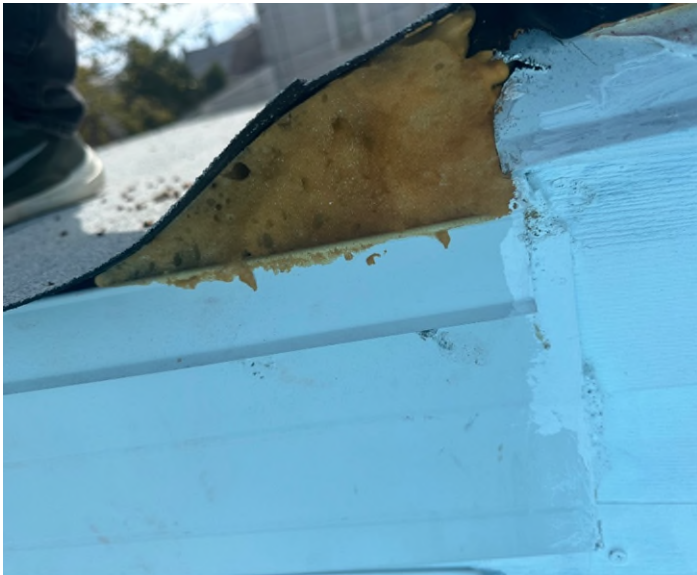
Current Roof (Applicant)
