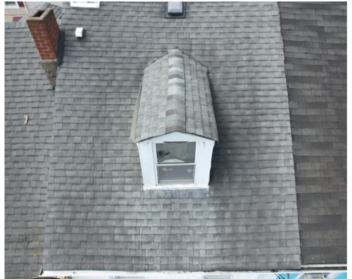
Current Roof (Applicant)
