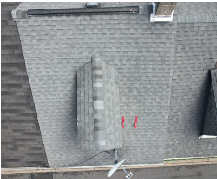
Current Roof (Applicant)
