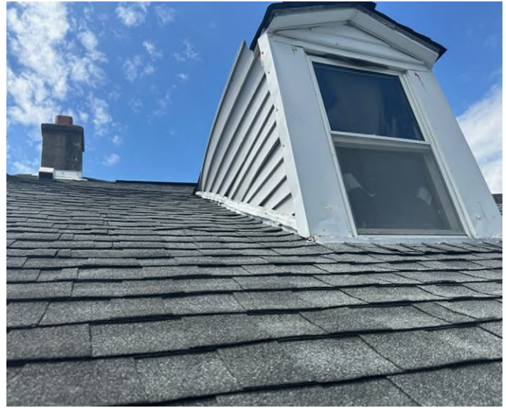
Current Roof (Applicant)
