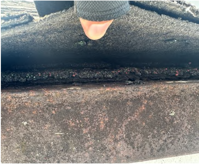
Current Roof (Applicant)
