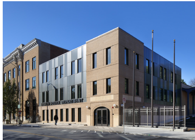
ABOVE: NEW EASTON POLICE STATION, 2016 - ALLOY5 ARCHITECTURE
