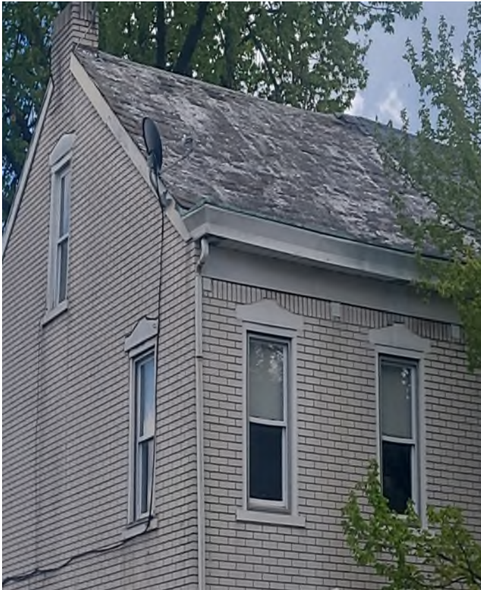
Current Roof (Applicant)
