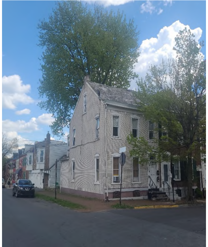
Current Roof (Applicant)
