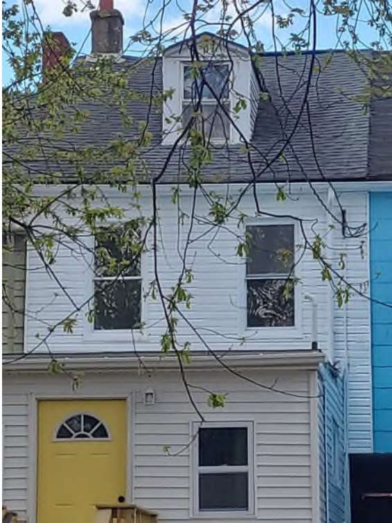
Current Roof (Applicant)
