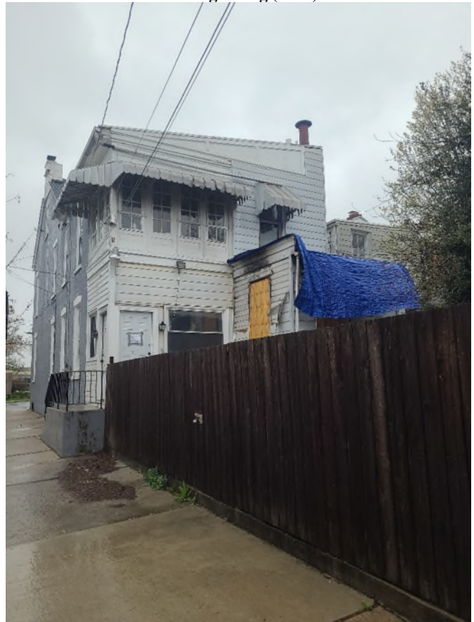
Existing Siding (Staff)
