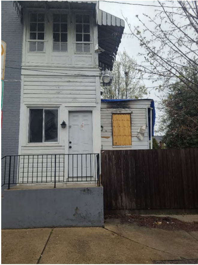
Existing Siding (Staff)
