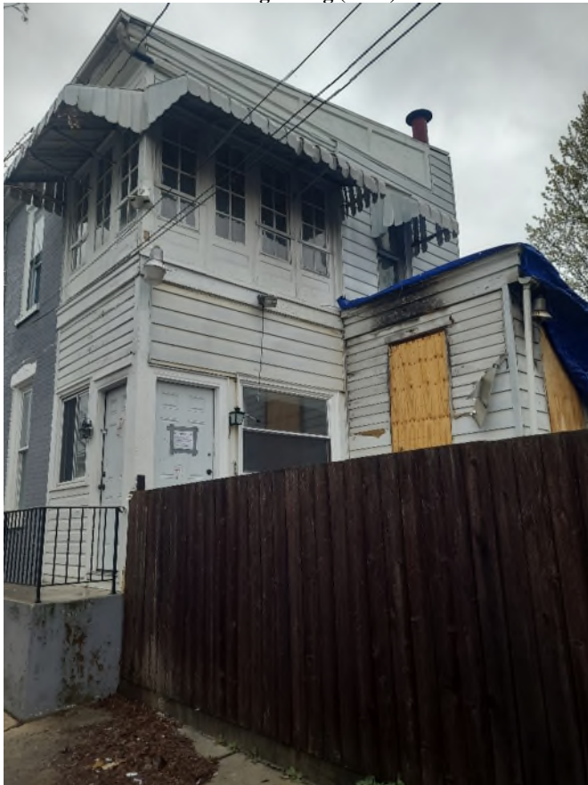
Existing Siding (Staff)
