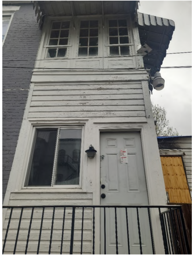
Existing Siding (Staff)
