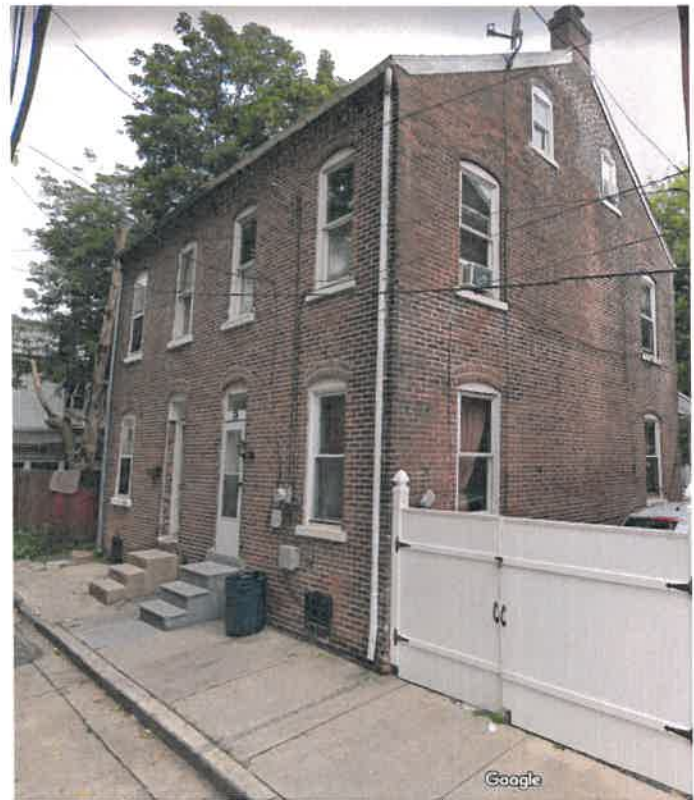
Front and side of 735 Oak Street, 2019. (Google StreetView)
