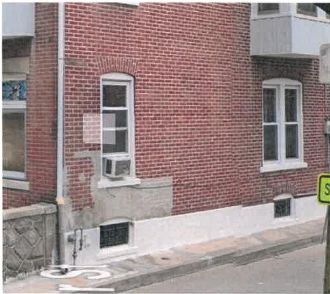
Poplar Street elevation of 1118 W. Turner Street, 2019. (Google StreetView)
