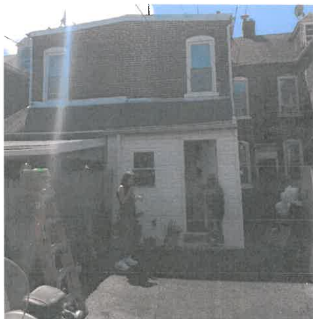
Rear of 937 North Street, 2023. (Applicant)
