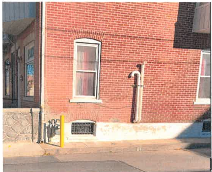
PVC pipes installed at 1118 W. Turner Street, November 2022. (Staff)
