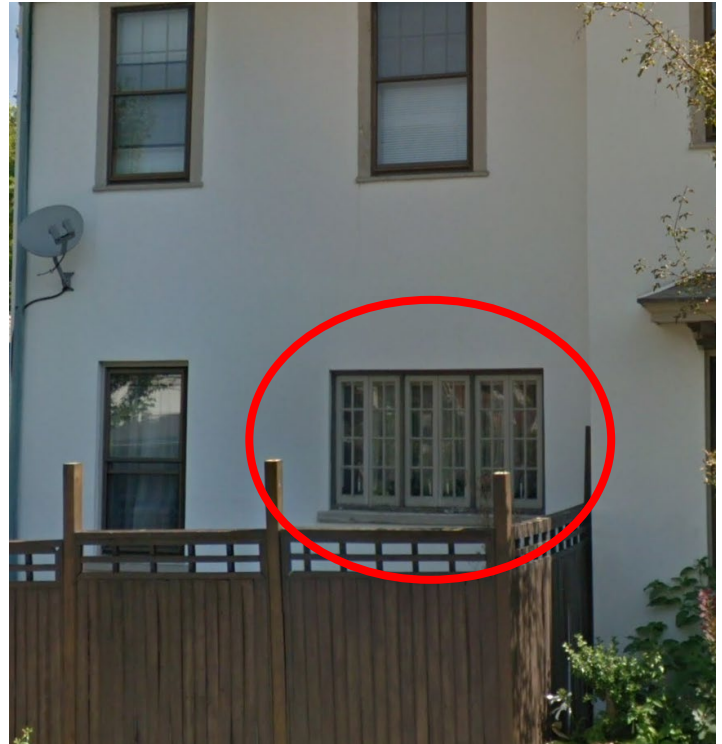
Side façade of 1625 W. Linden Street with the historic window circled in red, 2016. (Google StreetView)
