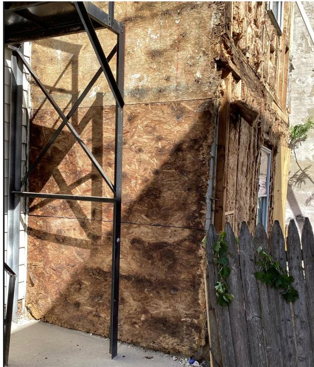
**Photo showing the wall condition following stucco removal.
