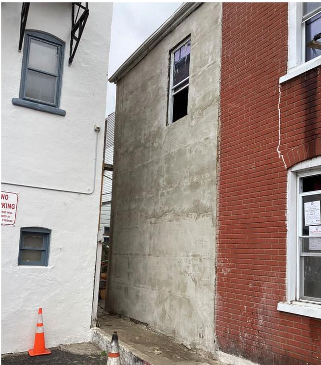
Photo showing rebuilt wall with door moved.
