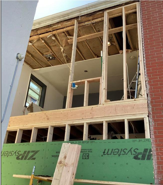
Side façade with walls removed and reframed.
