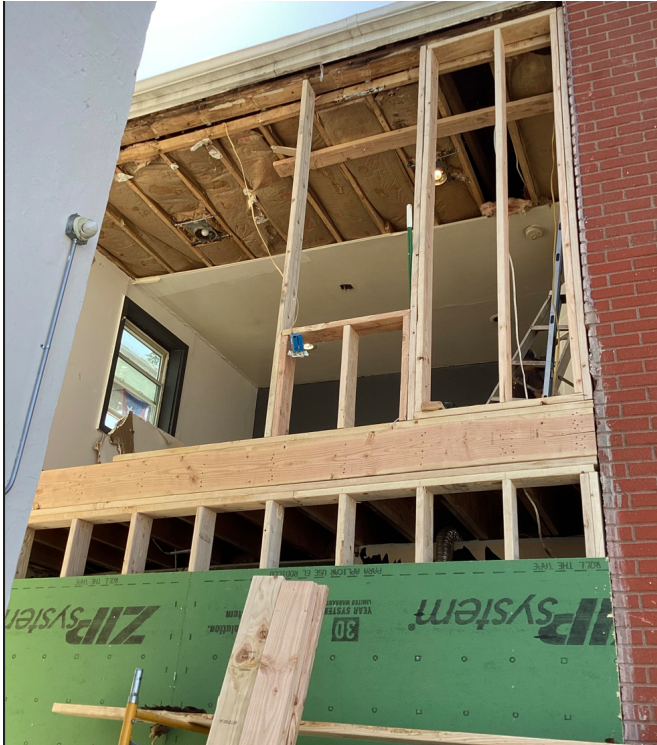
Side façade with walls removed and reframed. (City of Allentown)
