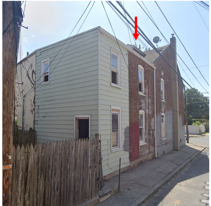
View of rear from Morris Street prior to removal, 2023. (Google StreetView)
