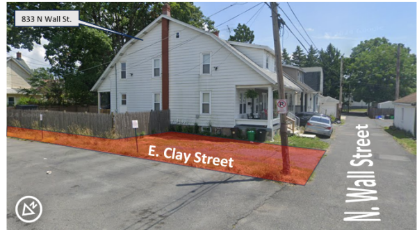
Figure 2 Street view of improvised parking and fence enclosure.
