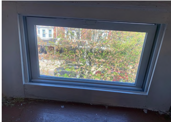
Installed Third Floor Window (Applicant)
