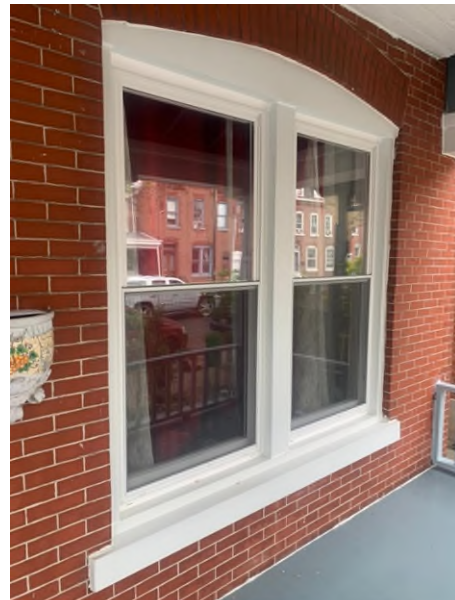
Installed First Floor Windows (Applicant)
