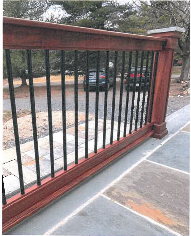
Proposed wood and metal railing. (Applicant)
