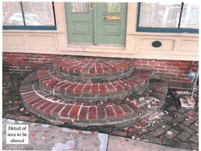
Existing steps at 346 N. 8th Street. (Applicant)
