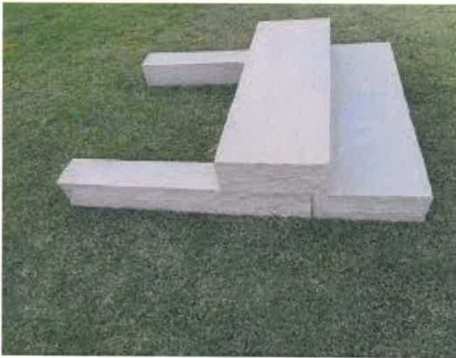
Partial construction of stone steps showing construction method. ( https://clsupplies.com/product/granite-fillers/ )
