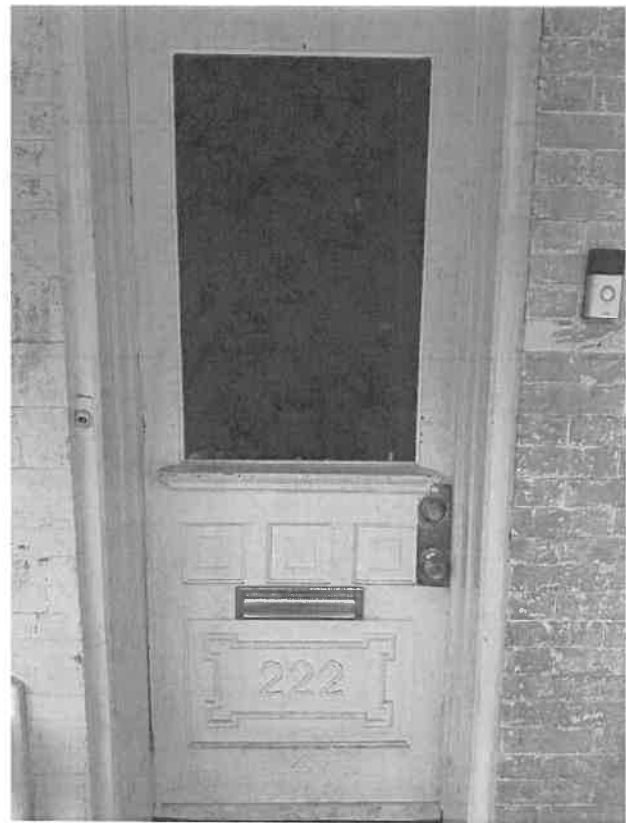
Existing Door (Applicant)
