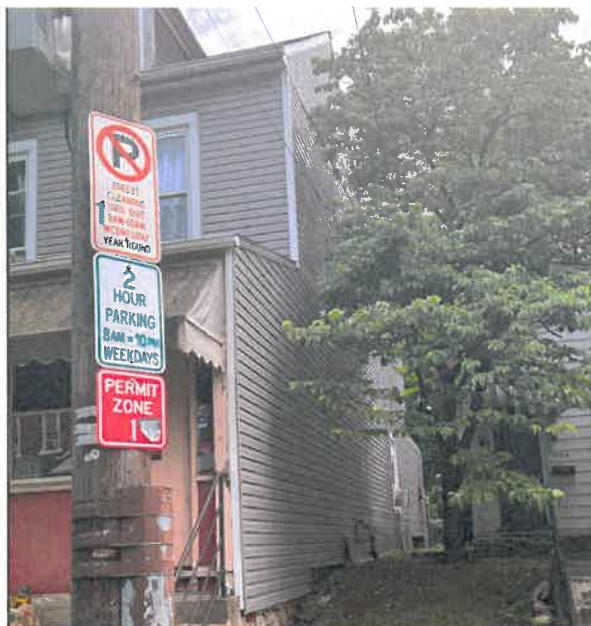
Side façade after siding was installed, 2023. (applicant)
