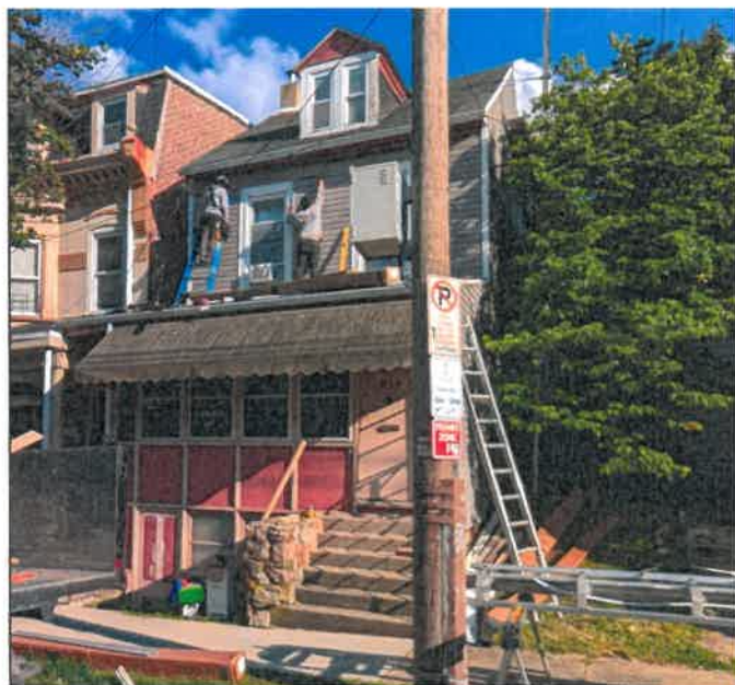
Front façade showing vinyl siding being applied, 2023. (HARB files)
