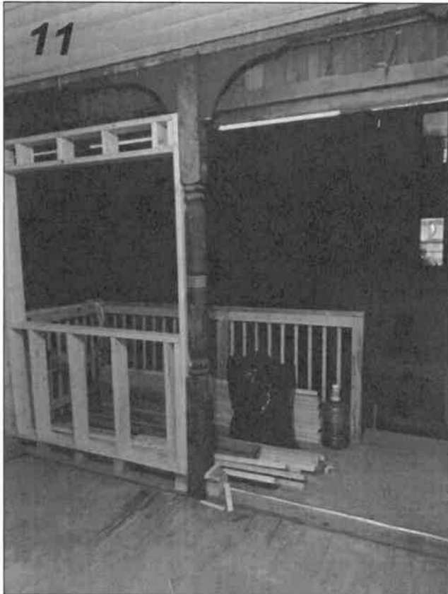
Process Photograph (Applicant)
