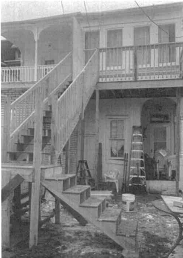
Existing back elevation (Applicant)
