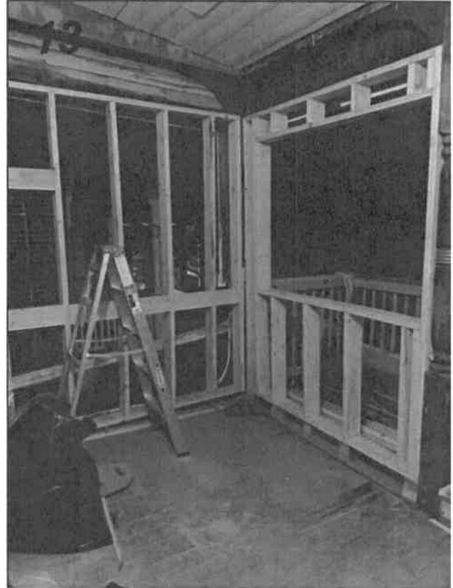
Process Photograph (Applicant)
