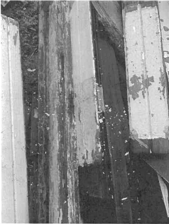
Rotted wood replaced (Applicant)
