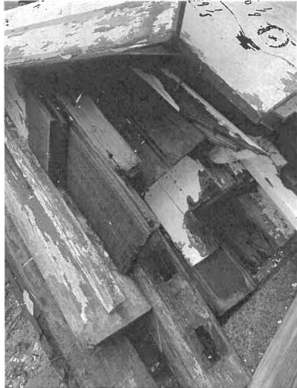
Rotted wood replaced (Applicant)
