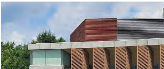
Mechanical equipment must be blocked from view on Primary Facades using walls and screens.
