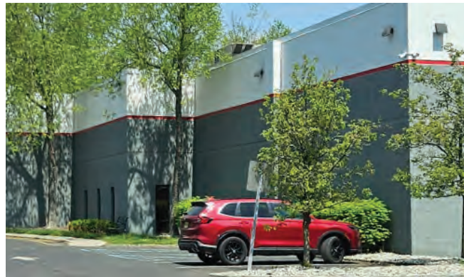
The cap shall have a change in material, color, and/or a projection. Primary Façades must have with visual vertical breaks at a minimum of 75' of horizontal length.
