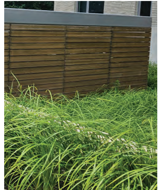
Decorative screen walls provide eight feet (8') or higher screening around three sides of the Ancillary Equipment.
