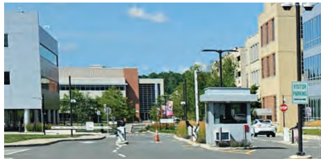
PIRT facilities with multiple buildings should be designed as a campus with shared amenities and open space
