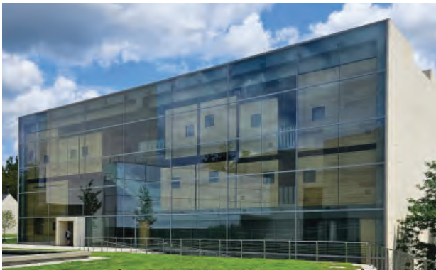
Primary Facades on Data Centers are to comply with all base design requirements in the PIRT District Design Guidelines.
