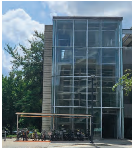
Main building entries shall project and/or feature a change in building material.
