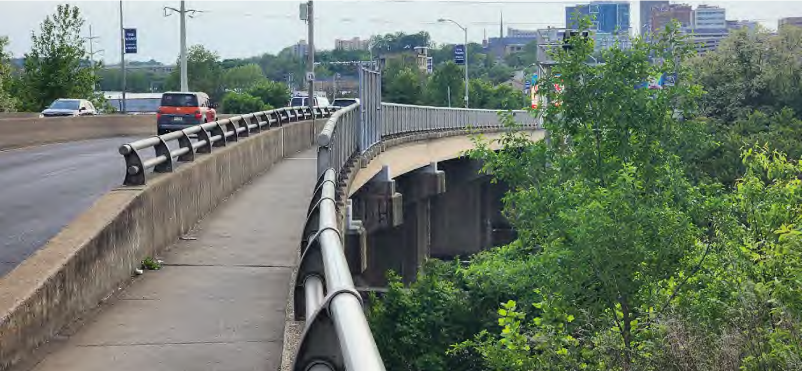
Hamilton Street Bridge over the Lehigh River
