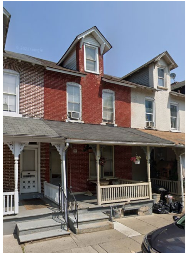
621 W. Liberty Street prior to reroofing, 2021. (Google StreetView)
