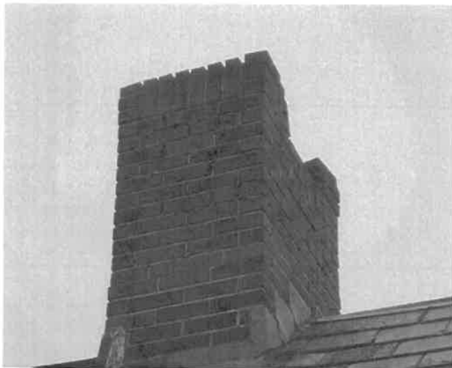
Current Chimney (Applicant)
