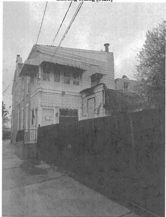
Existing Siding (Staff)
