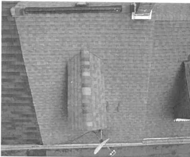
Current Roof (Applicant)
