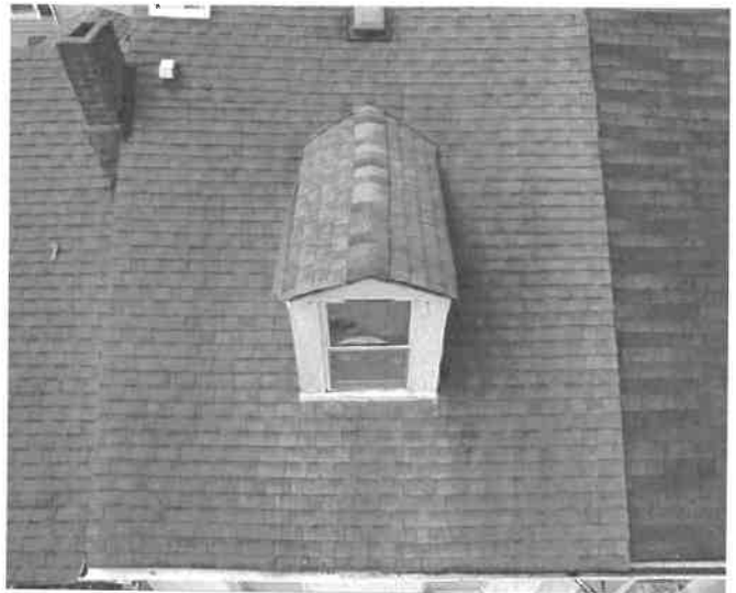
Current Roof (Applicant)
