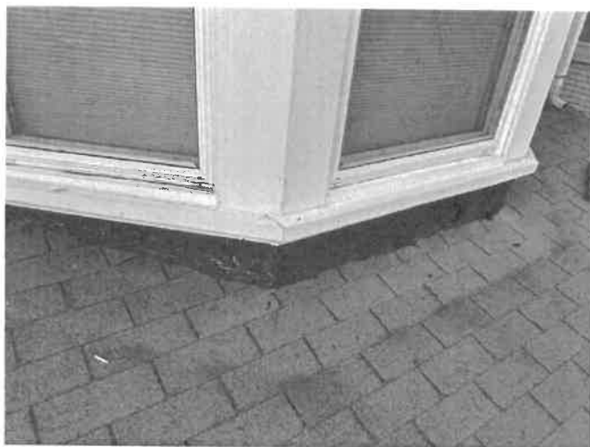
Roofing at Bottom of Bay Window (Applicant)
