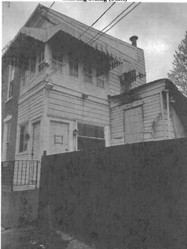
Existing Siding (Staff)
