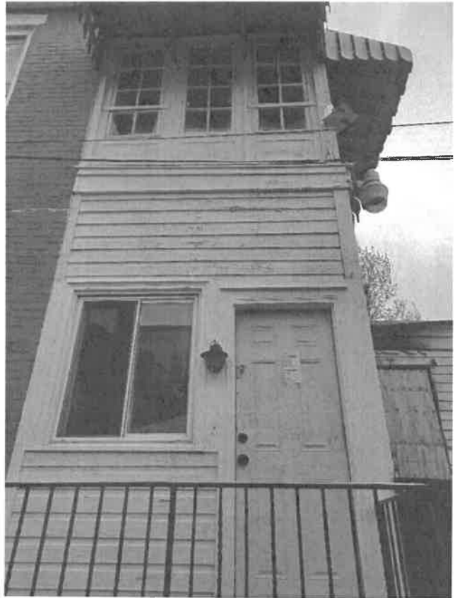
Existing Siding (Staff)
