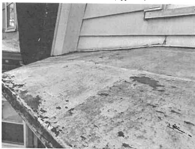
Bay Window Roof (Applicant)
