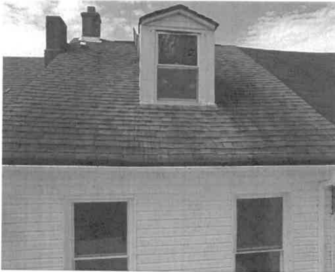
Current Roof (Applicant)
