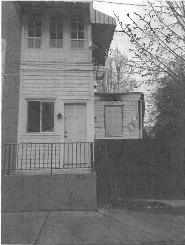
Existing Siding (Staff)
