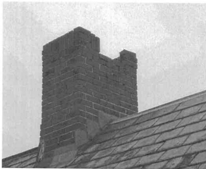
Current Chimney (Applicant)
