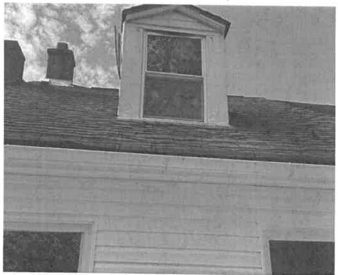
Current Roof (Applicant)
