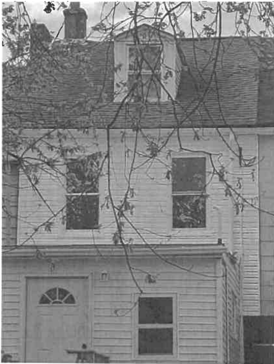
Current Roof (Applicant)
