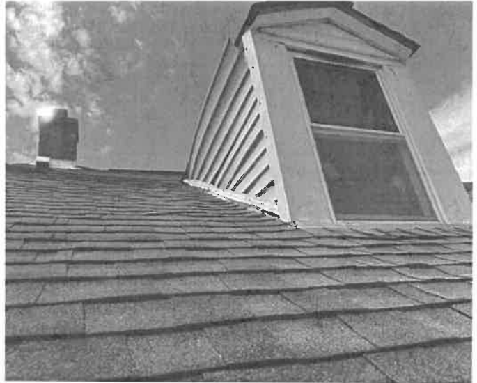
Current Roof (Applicant)
