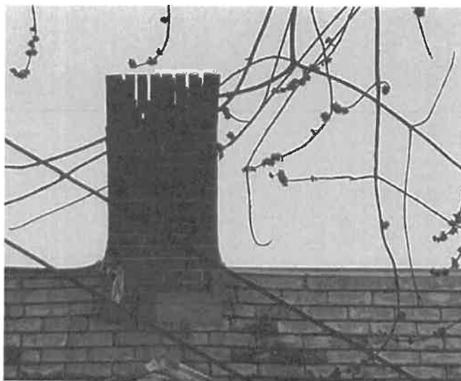
Current Chimney (Applicant)
