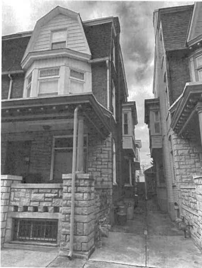
Front Facade (Applicant)
