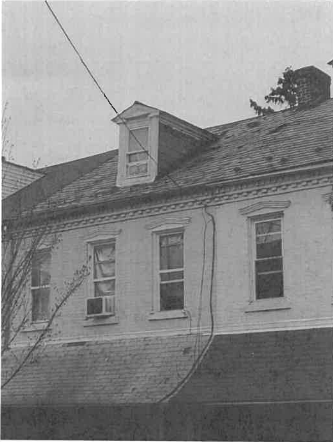
Current Roof (Applicant)
