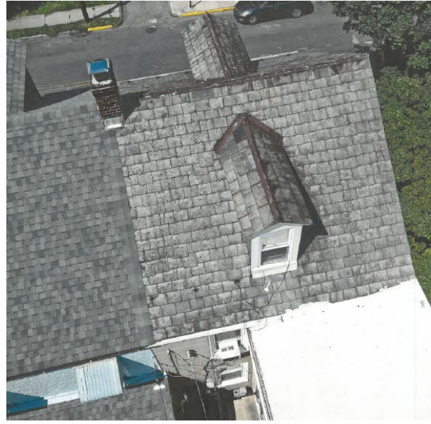
Back Roof Aerial of 213 N. 11 th Street, 2023. (Applicant)
