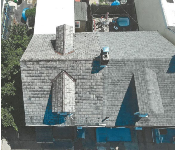
Front Roof Aerial of 213 N. 11th Street, 2023. (Applicant)
