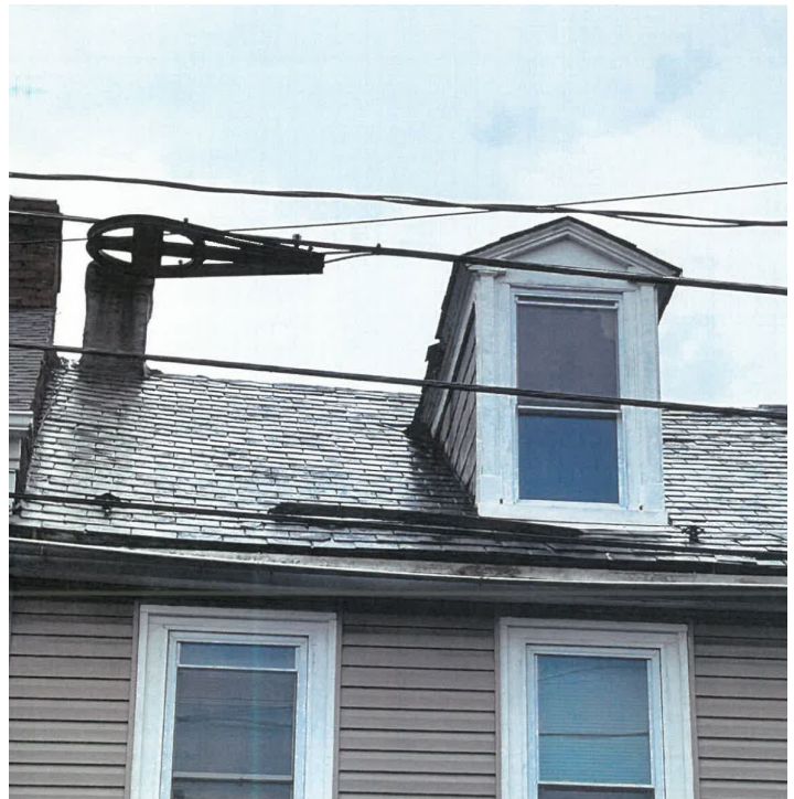
Detail of roof, 2023. (Applicant)
