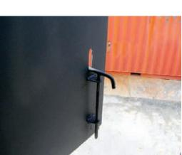
Figure C-6: Window & Latch Construction
