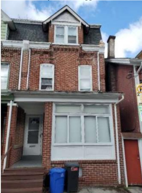
Primary Facade (Applicant)
