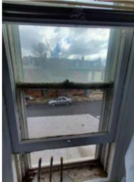
2 nd Floor Front Window (Applicant)
