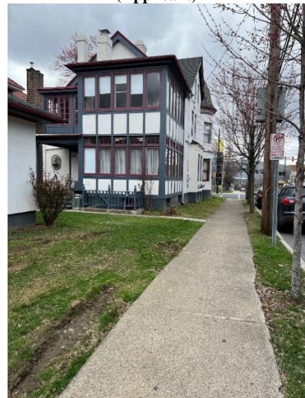
Rear facade, view from Linden St. (Applicant)
