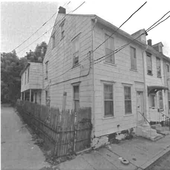
The main structure of 948 North Street in 2019. (Google StreetView)
