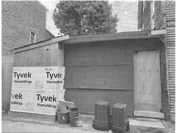
Existing condition of rear ell facing Refwal Street. (Applicant)
