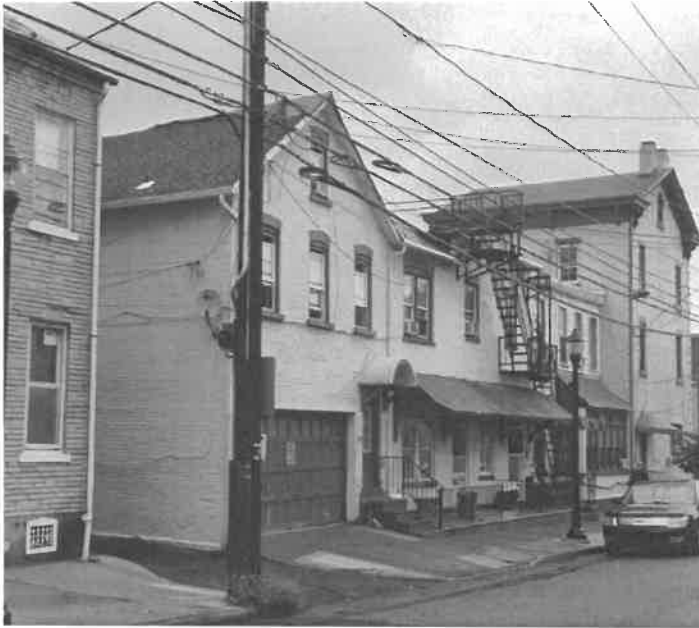
402 N. 6th Street showing gable roof replacement, September 2022. (Applicant)
