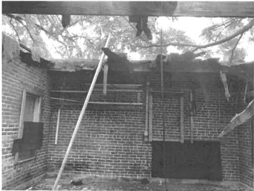
Interior of the garage at 948 North Street. (Applicant)
