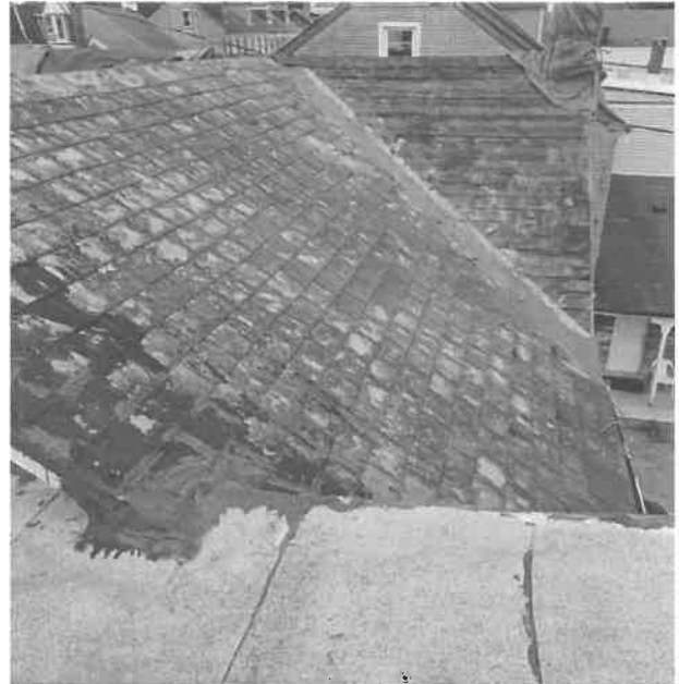
402 N. 6 th Street remaining slate. (Applicant)
