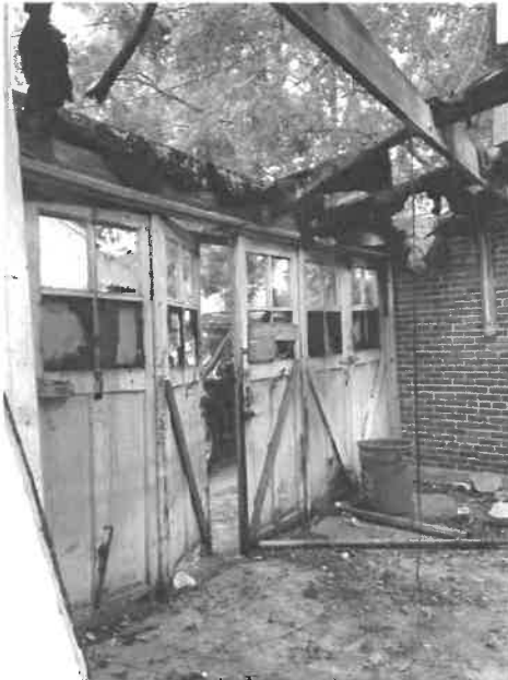
Interior of the garage at 948 North Street. (Applicant)
